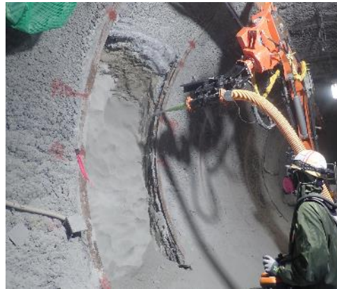
Excavation Damage Zone (EDZ) identification and sealing test
