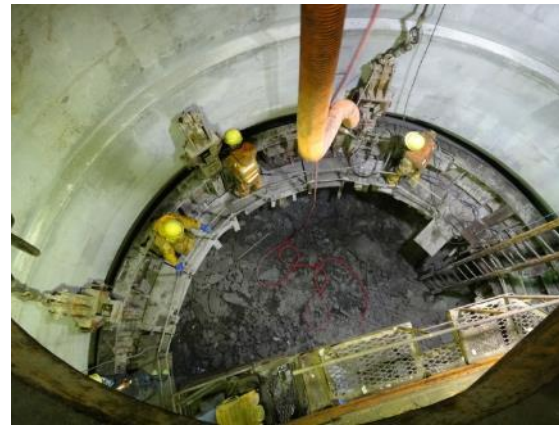
East Access Shaft
