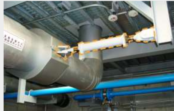
Seismic reinforcement of piping
