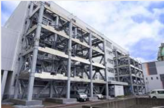
Seismic reinforcement of administrative offices
